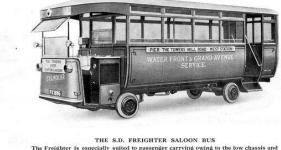
The Freighter is especially suited to passenger carrying owing to the low chassis and smooth riding. The above shows one of a fleet of Preighter Buses in service on the South Coast.
