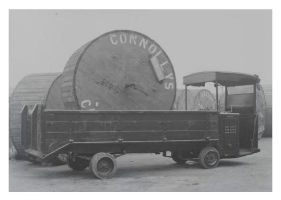
Standard cable drum lorry. Complete with winches and drum chocks. 12 ft. X 6 ft. X 2ft. Load 3 tons
