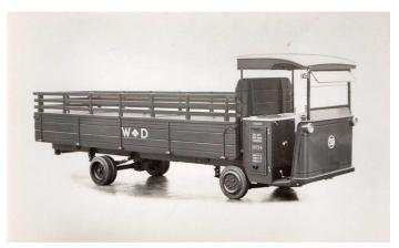
Factory truck. Steel deck and timber sides. 9 ft. x 4 ft. 9 ins. x 1 ft. 6 ins. Load 2 TONS. Price: £482 10s. 0d.
