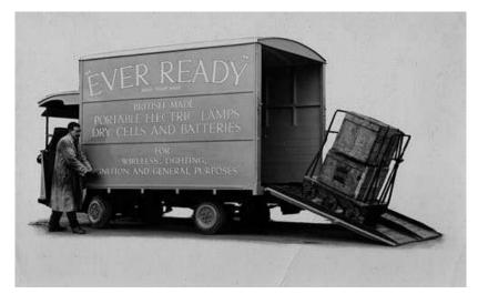
BOX VAN WITH WINCHES AND RAMP END. 10 ft. x 6 ft. 6ins. LOAD 2 tons. Price £640 **Photo supplied by Malcolm Easton.**
