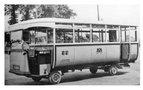
This picture shows one of the six Freighters operated by Plymouth Corporation under the transport manager of the time, H P Stokes. The first three (numbers 22-24) had Hickman bodies and were introduced in June/July 1922 and the second three (numbers 45-47) had similar Vickers bodies and arrived in May 1926. All six were withdrawn and sold in 1929/30.
