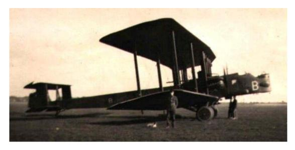
The above photograph is of a Vickers Virginia biplane heavy bomber developed from the Vickers Vimy for the Royal Air Force, The first squadron of Mark I Virginias was assembled in 1924. Despite mediocre performance, the aircraft served frontline units until 1938, when it was replaced by the newer Wellingtons, Hampdens and Whitleys. The photo shown below appears in Kaleidoscope of Shelvoke & Drewry as Caption 85.
