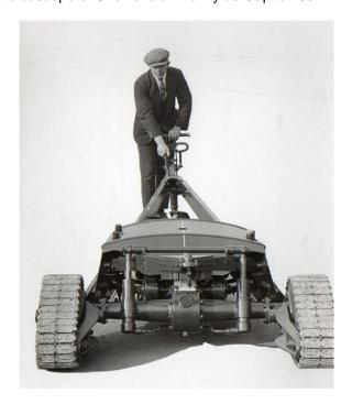
The caption informs us that the R.A.F. were supplied with twenty-nine of these trolleys between 1929 and 1933 for ground handling of the Vickers Virginian bombers. Powered by a flat four air cooled petrol engine and with epicyclic transmission hydraulic rams raised a towing pin which connected with a ring on the aircraft and permitted one man to tow or turn the bomber with ease.
