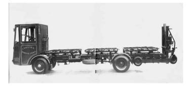
Other Councils adopted similar methods of refuse collection especially from blocks of flats and the above photo shows an SD 'W' type equipped to carry three wheeled containers for the London Borough of Chelsea.
