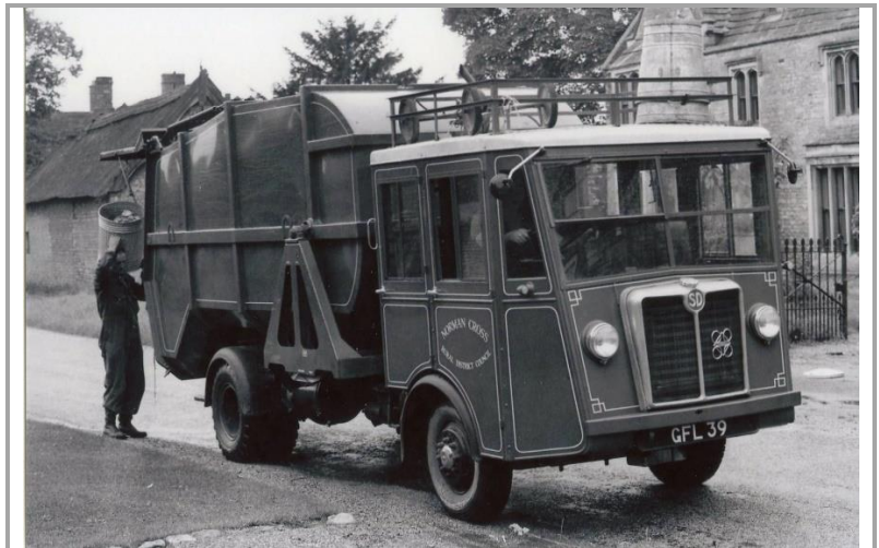
Above:- Around 1948 the 'W' type became available with a Fore & Aft tipping body. This is a later version fitted with a Perkins diesel engine which could be specified from 1954.
