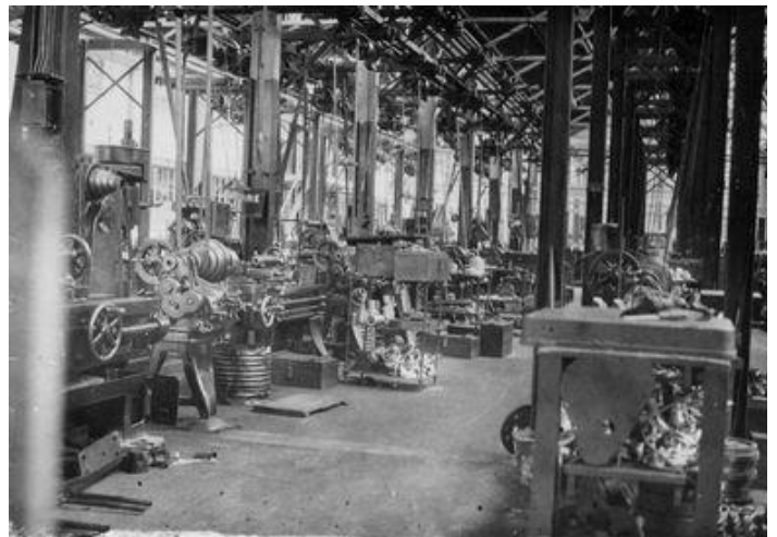
The Machine Shop. Note:- The machines are belt driven from a shared motor.
