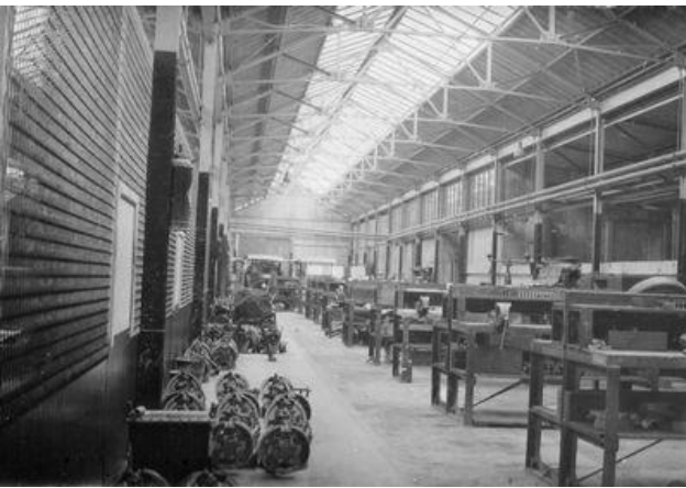
On the left of the photo completed axles assembled on the right hand benches
