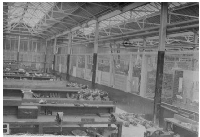
Another view of the sub-assembly benches.
