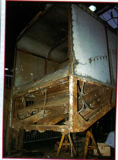
Not a pretty sight! All the corroded areas were replaced.
